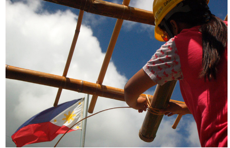
a student wraps uway (rattan) around bamboo joints
